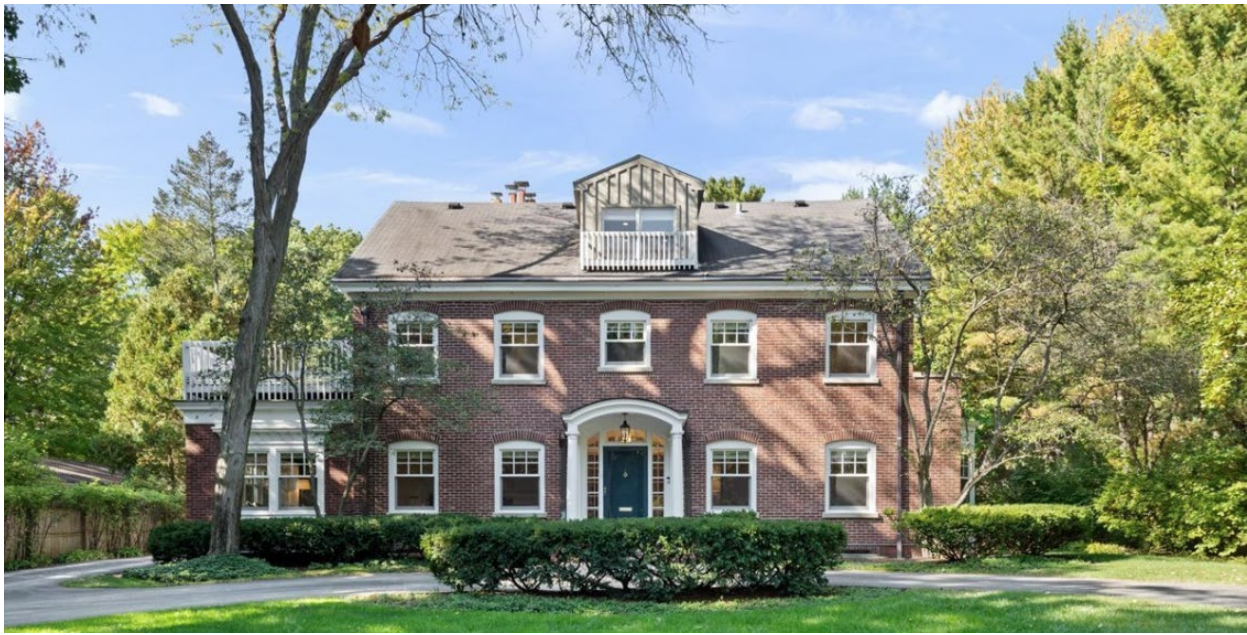
Figure 1. Front Façade, Dec. 2025, credit Baird and Warner.
