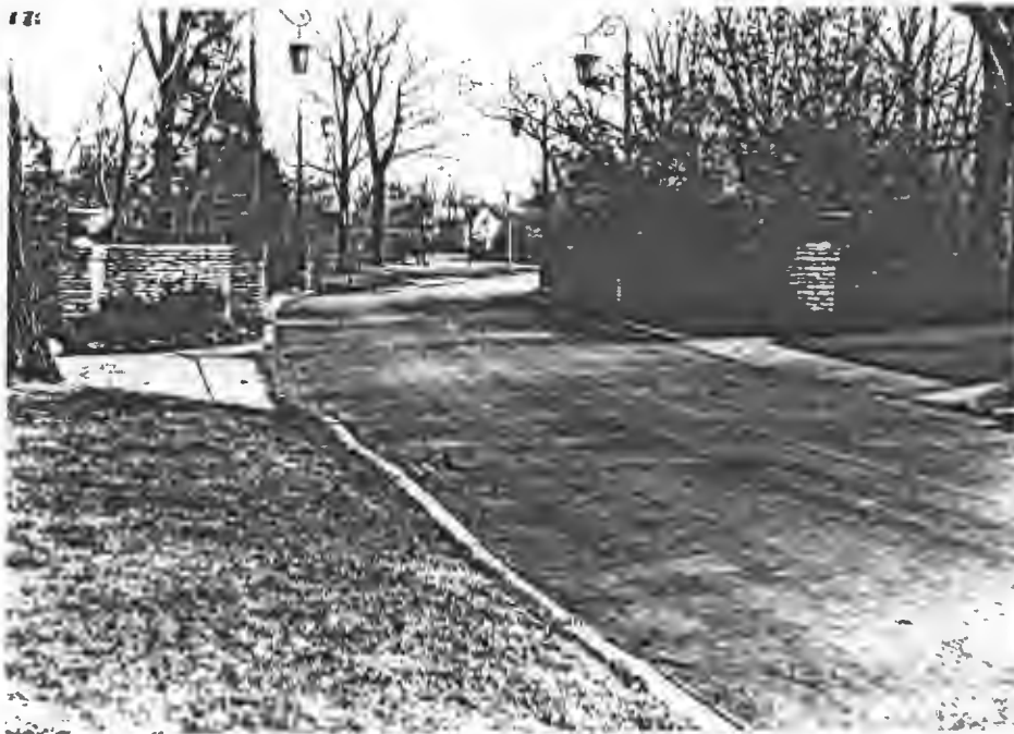
Jensen bridge on S. Deere Pk
