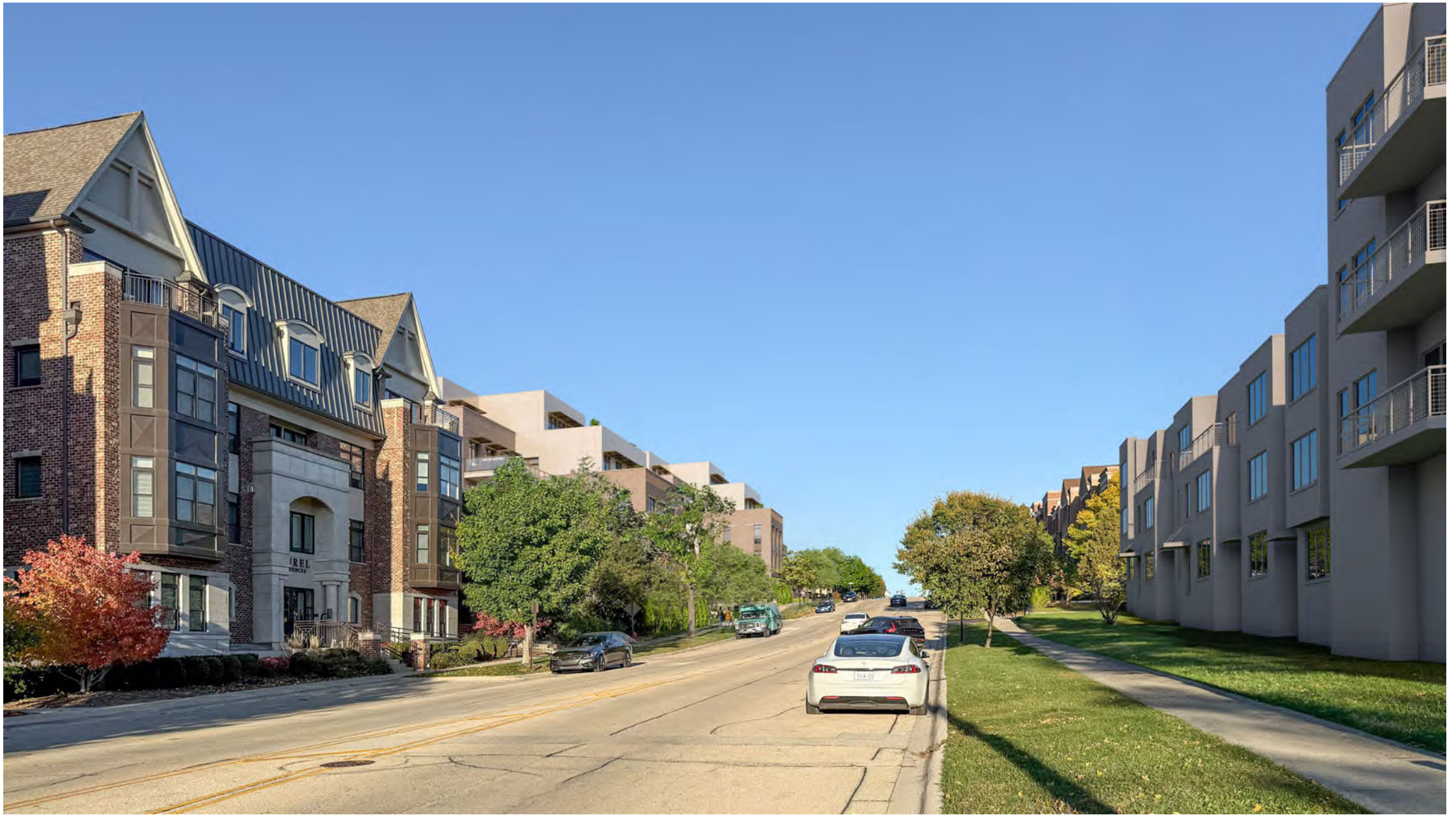
VIEW LOOKING EAST UP LAUREL AVENUE
