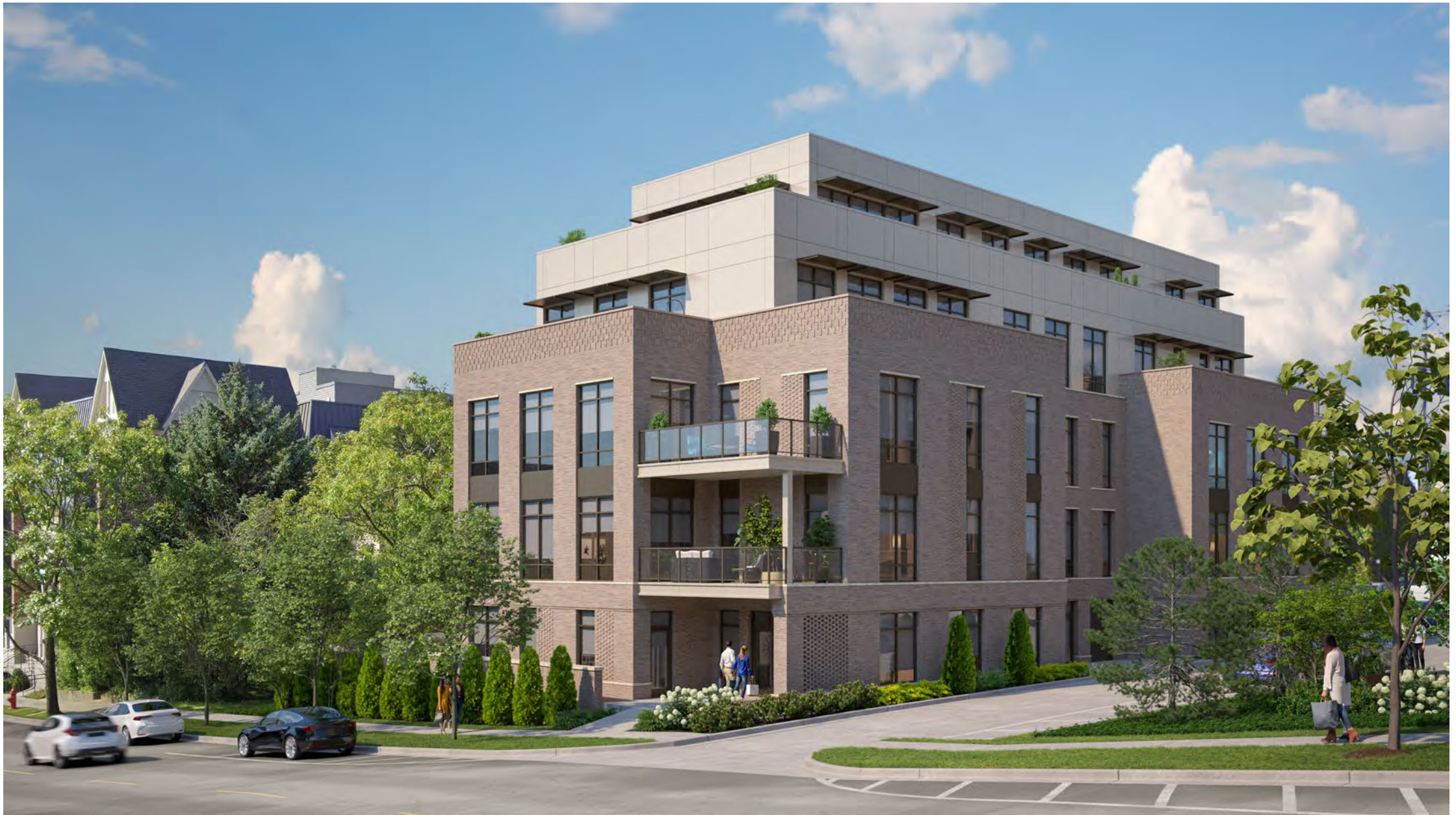
VIEW OF WEST BUILDING AND ALLEY FROM LAUREL AVE
