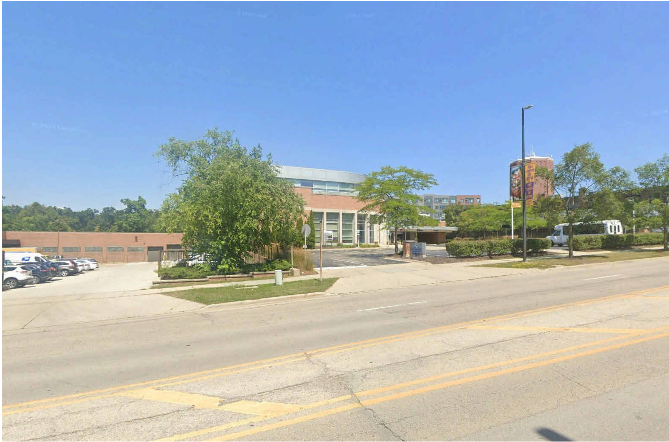
FROM CENTRAL AVE LOOKING NORTH
