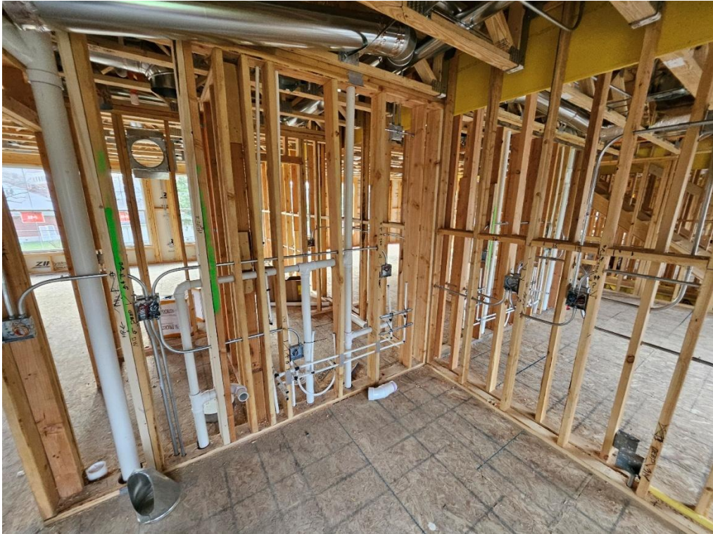
Typical Lower Level Laundry Room, HVAC, Electric, Sprinklers
