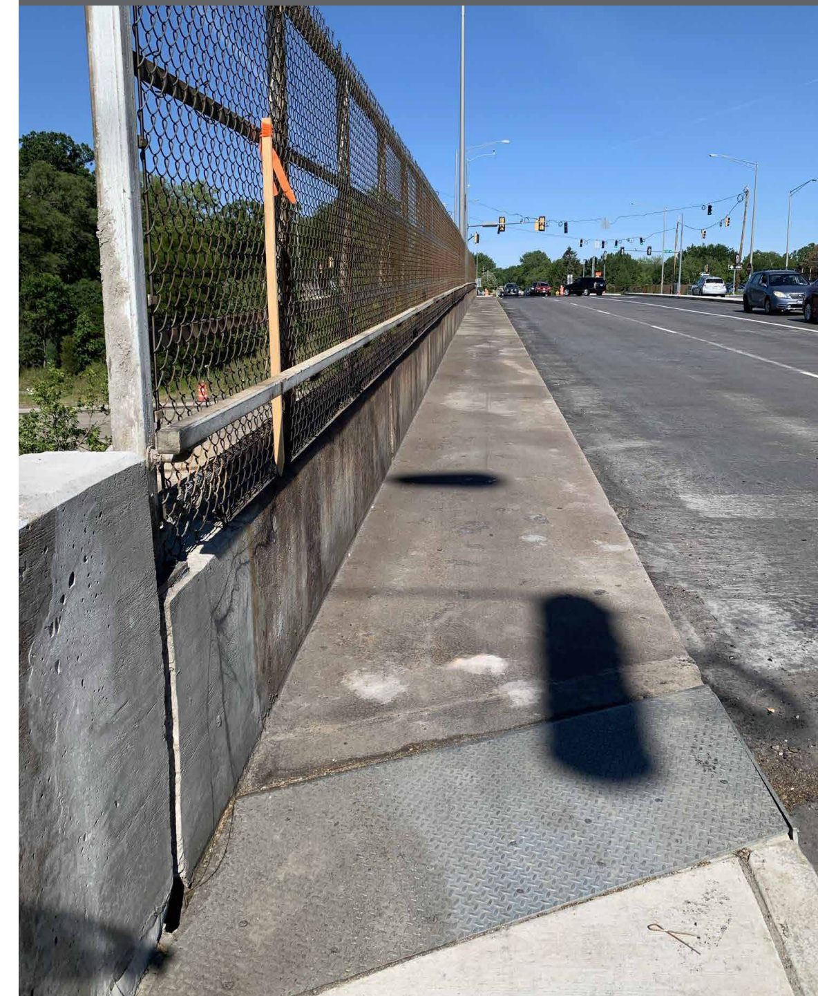
Looking east on the bridge over US-41.
