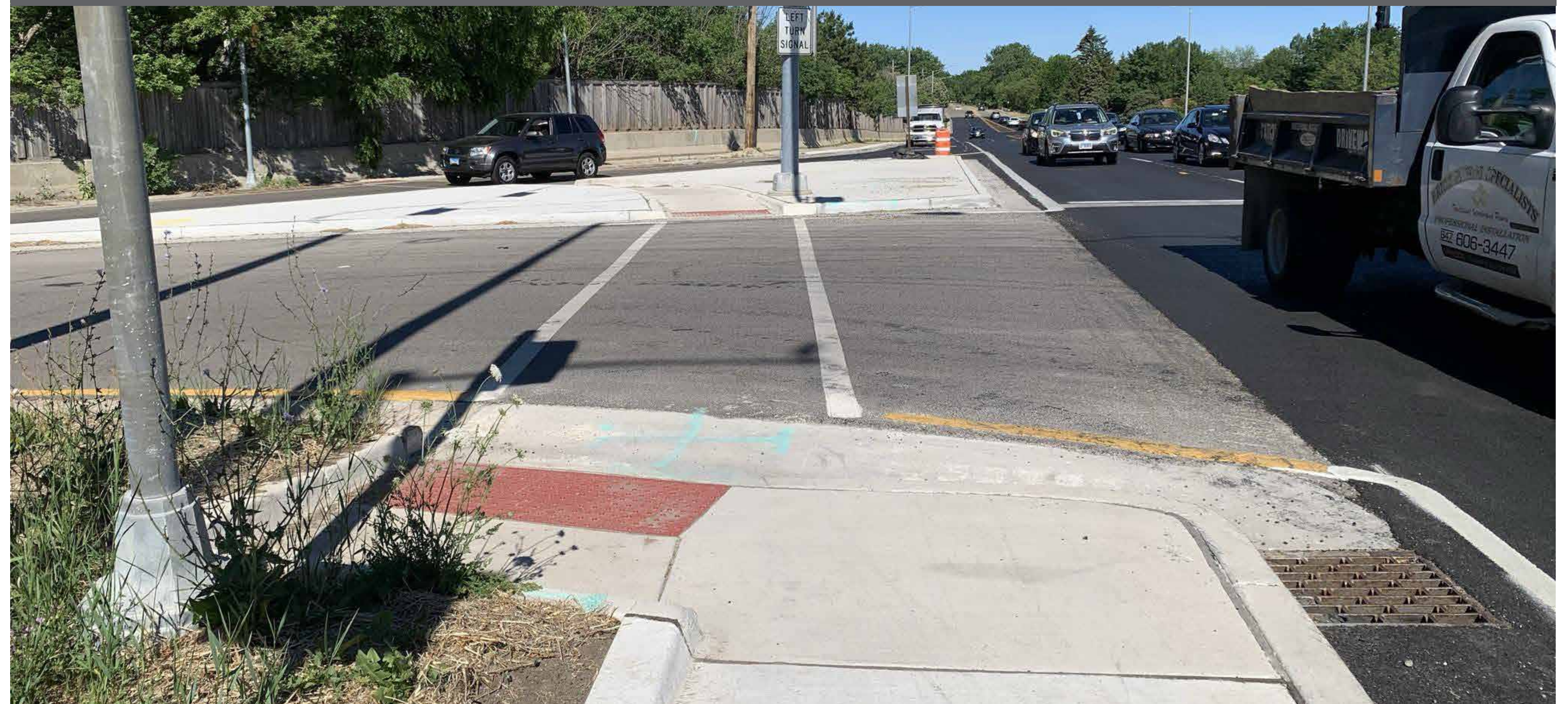
Looking east at the US-41 northbound on-ramp.
