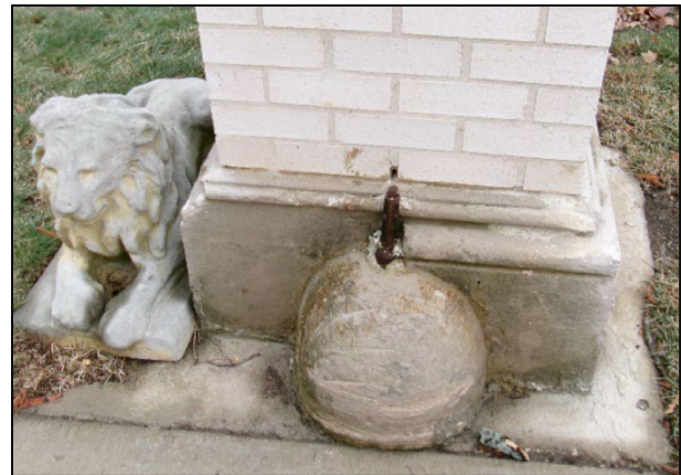
Figure 3. Wrought-iron remnant at base of gatepost
