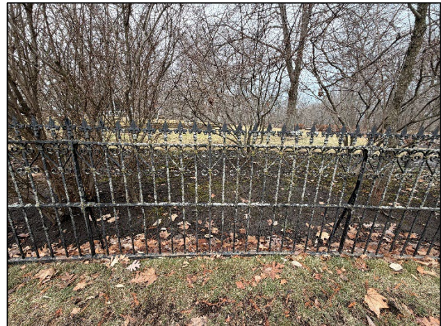
Figure 1. Historic fence located on proposed Lot B
