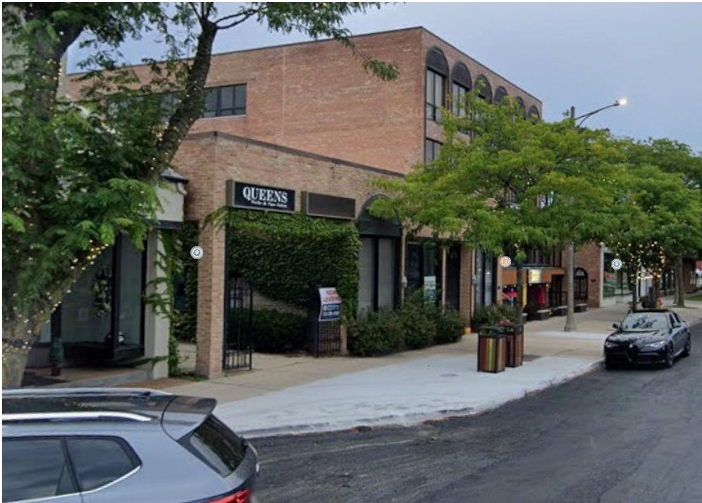
Looking North at Property
