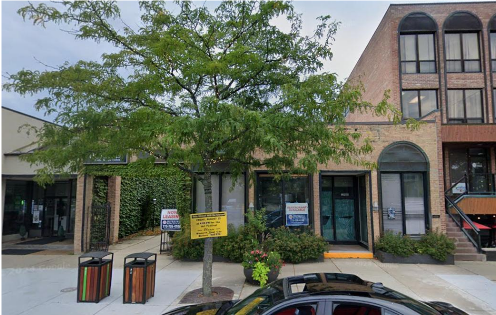
1900 First Street – Front Façade (looking west)
