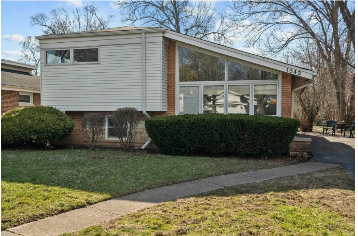
1342 Ferndale, Highland Park (During Rehab)
