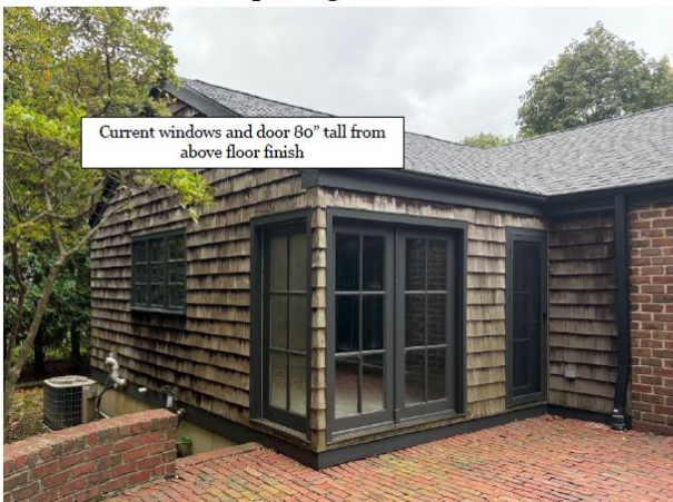
Current Kitchen Openings
