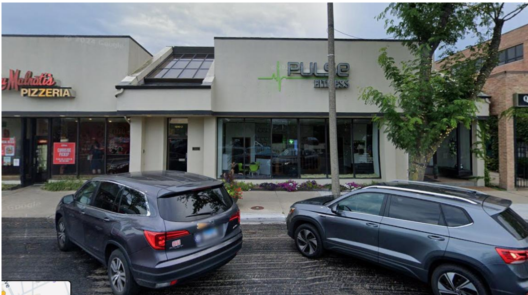
Property South (The Box – 1890 First Street)
