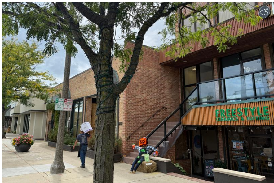
Looking South at Property
