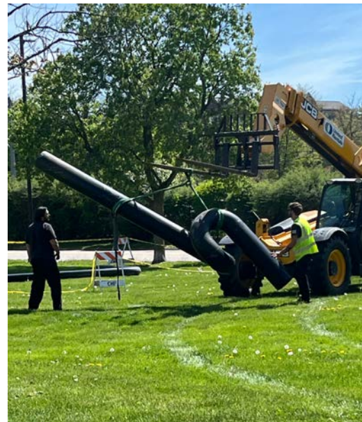
Moving the Sections With the Telehandler
