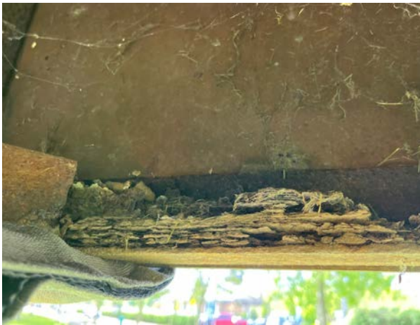
Jack Resting on Interior Structure
